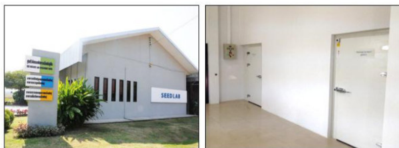
Figure 7 Cold storage room (Seed lab)
