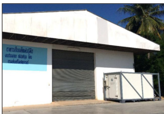
Figure 16 Container testing at Ni KhomLansak Cooperatives
